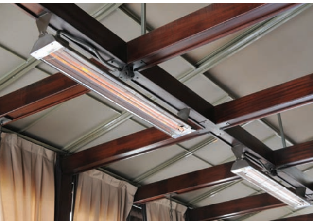
Restaurant with powder-coated bronze W-Series heaters ceiling mounted to a wood beam
